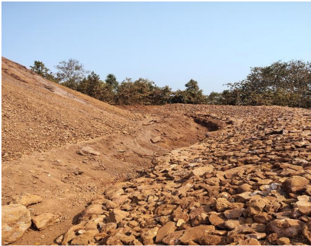
Photo-8 Retaining wall with garland drain at the toe of OB dump at Block II area
