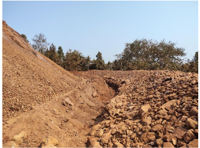
Photo-8 Retaining wall with garland drain at the toe of OB dump at Block II area
