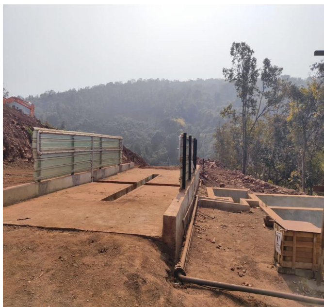
Photo-3 Wheel wash facility at the exit gate of Mines with recirculation system
