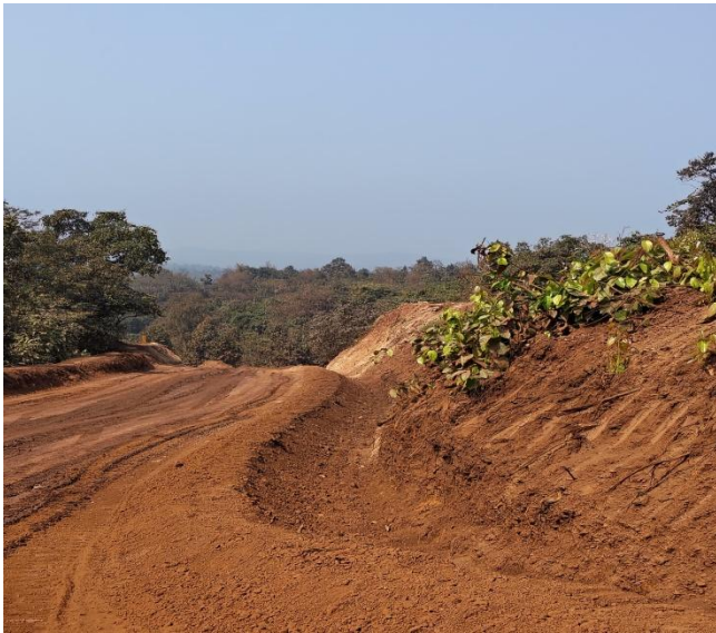
Photo-9 Garland drain at the toe of OB dump at Block II area
